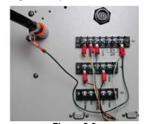
Figure 2-3 Installed Grounding Assembly
