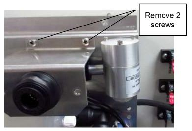
Figure 6-7 Remove inlet mounting screws
